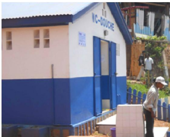
A WASH block constructed by WASHplus in the Nanisana area of Tana.
